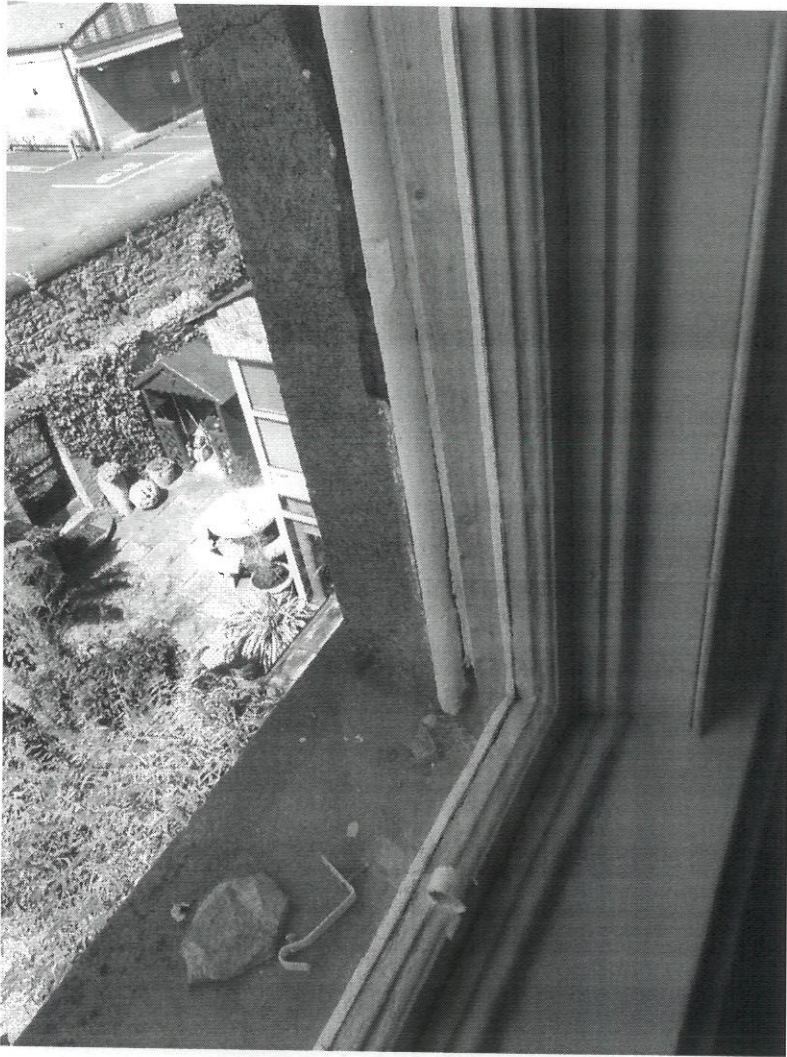
Photo 5 – Window to rear, note failing external reveal with debris on sill, and prop to upper sash (broken cords)
