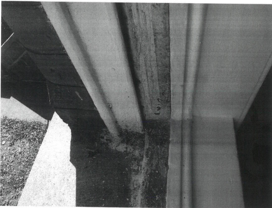
Photo 4 – Typical window sill to the front, generally good condition
